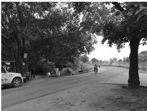
Figure 2: Sharp bends requiring curve warning sign and chevrons
