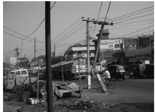
Figure 4: Broken poles, low height wire inviting danger
