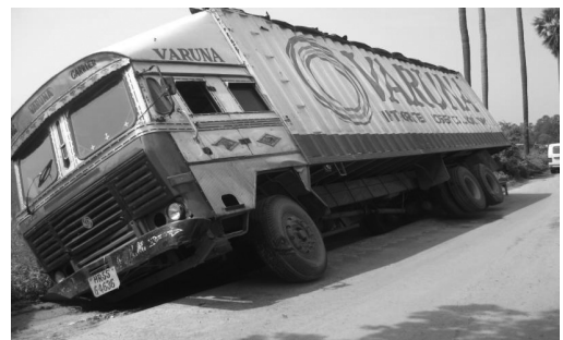
Figure 5: Inadequate earthen shoulder
